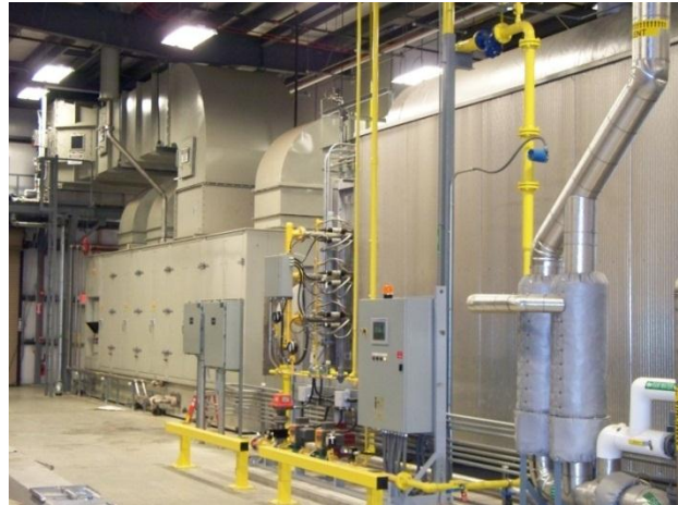
Figure 1. A typical 1.5 MW gas turbine CHP system
