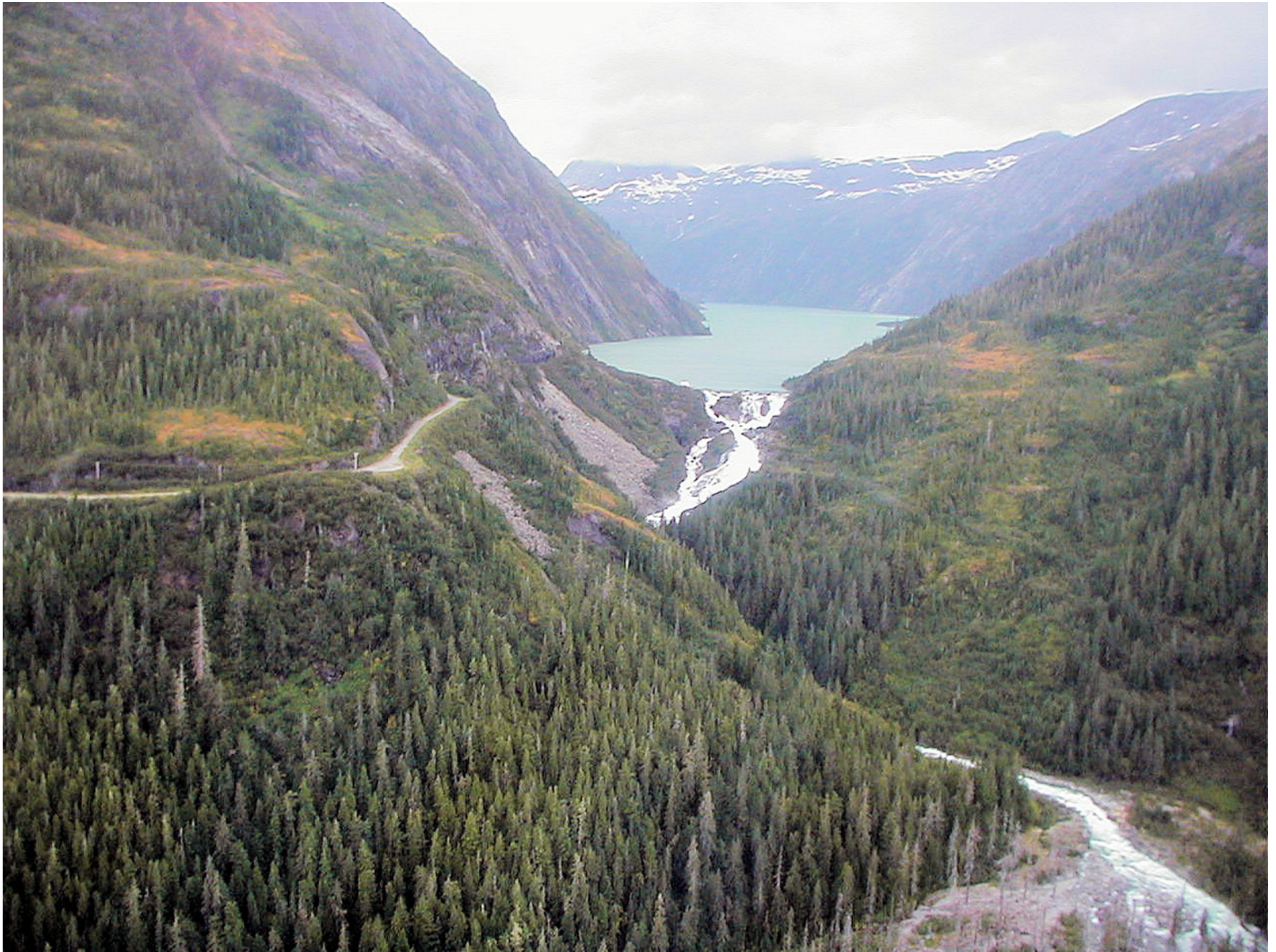
Long Lake, Snettisham Hydroelectric Project.
