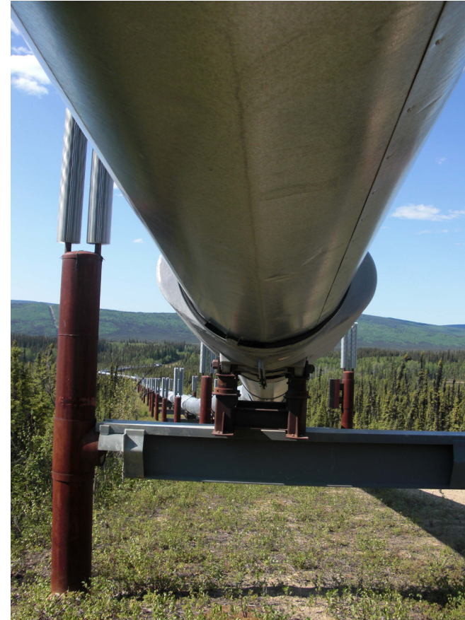
Trans-Alaska Pipeline at Fox, Alaska
