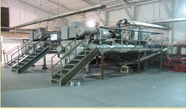
Above: The 400 kW geothermal power plant at Chena Hot Springs. Named the Chena Chiller. This unit is unique in that it is designed to work with geothermal fluids much cooler than any other plant.
