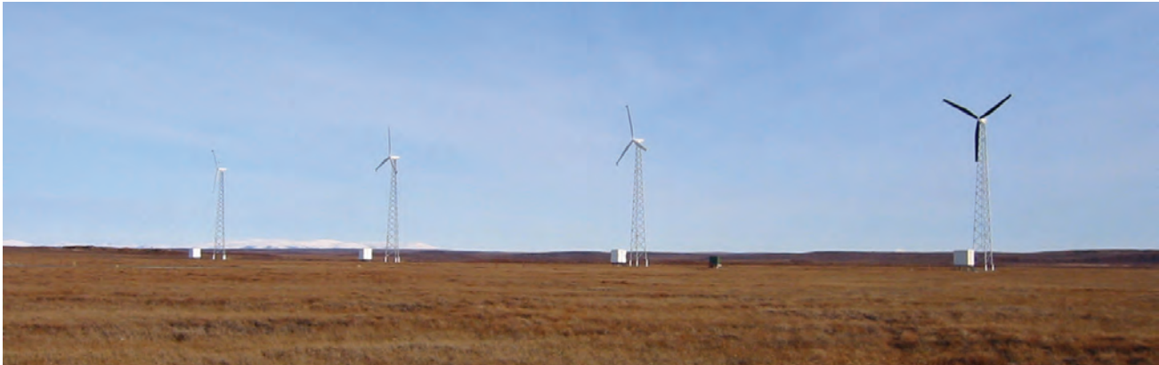
Four 66 kW Integrity wind turbines that make up part of Kotzebue Electric Association's 1,155 kW wind farm. In a typical year, the 17-turbine wind farm displaces over 100,000 gallons of diesel fuel.
