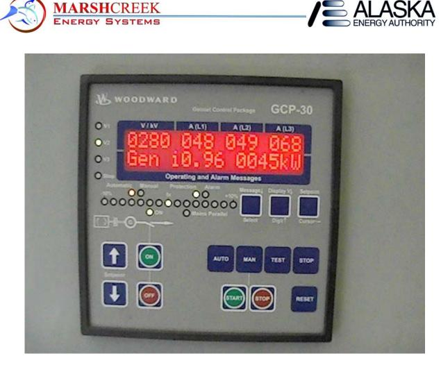
GCP-30 used in Stevens Village switchgear. Note the similarity in layout and design to the GSS offered by PowerCorp.
