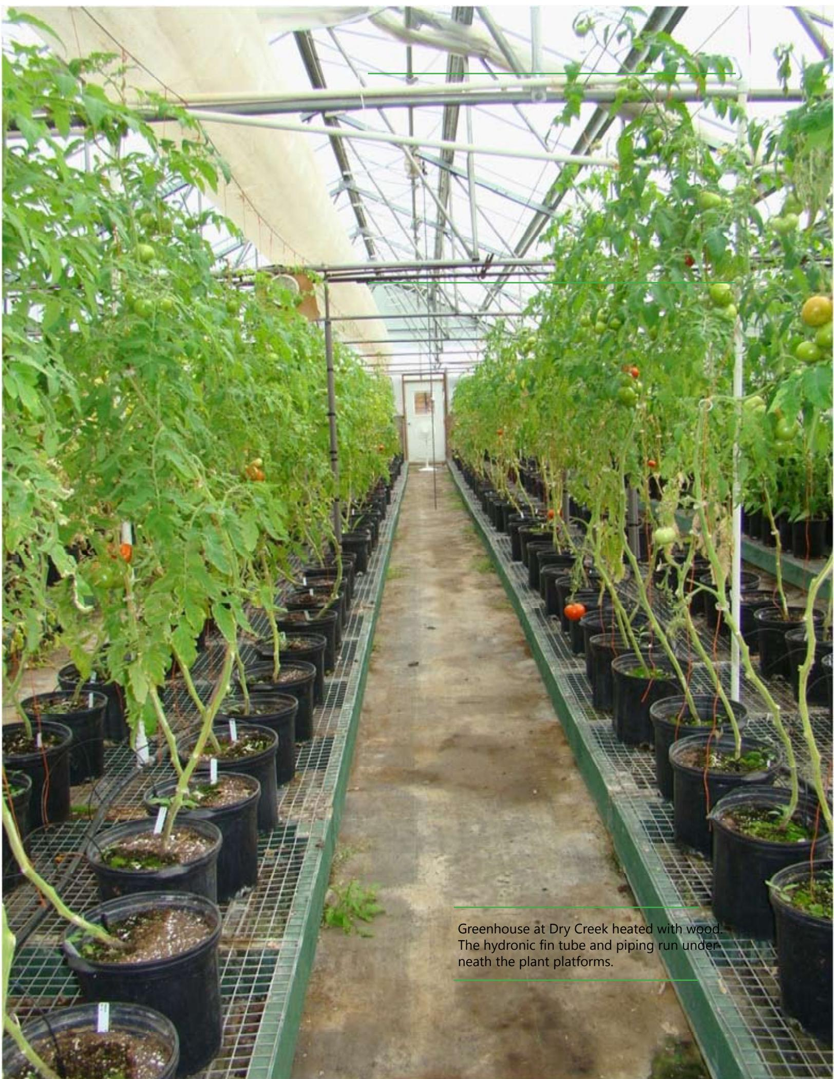
Greenhouse at Dry Creek heated with wood. The hydronic fin tube and piping run underneath the plant platforms.
