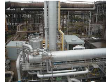
Steel Plant (Japan)
