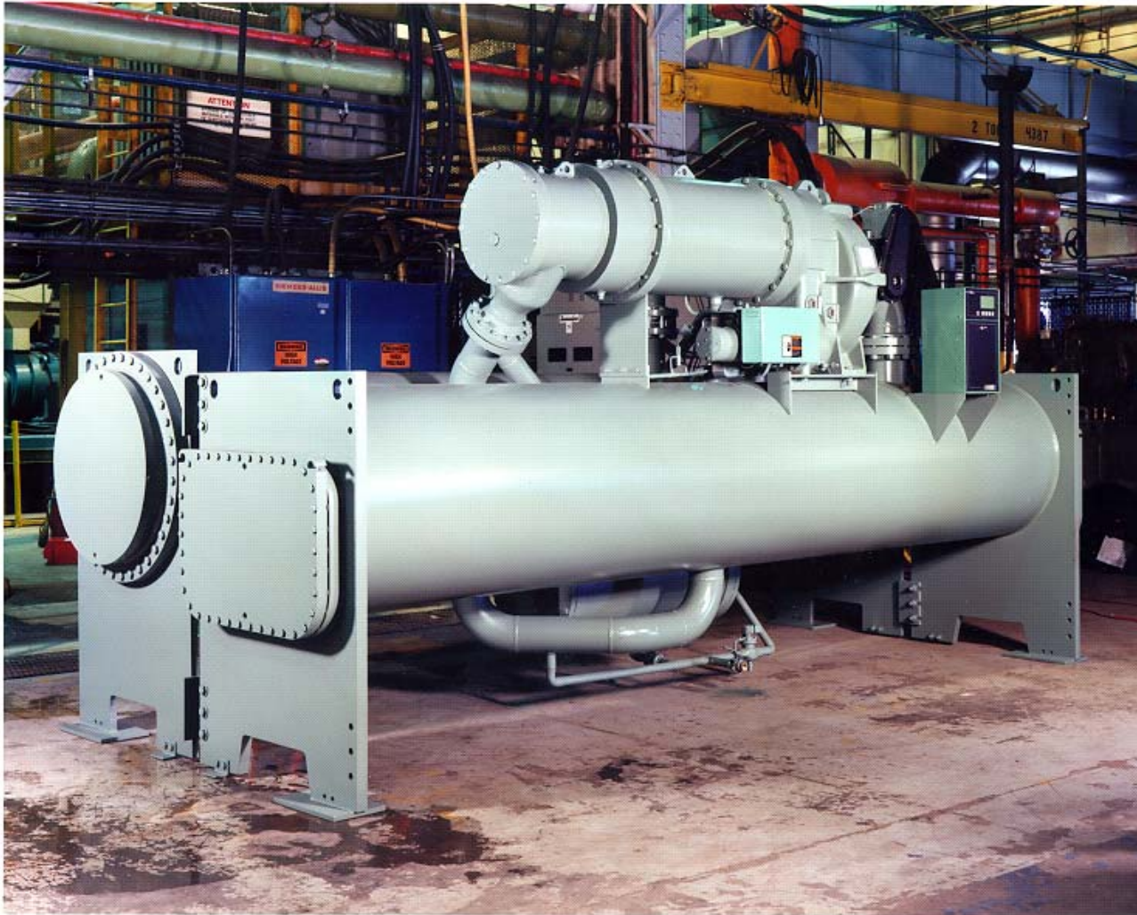
Figure 14 Commercial Chiller Incorporating Two-Phase Turbine for Energy Recovery
