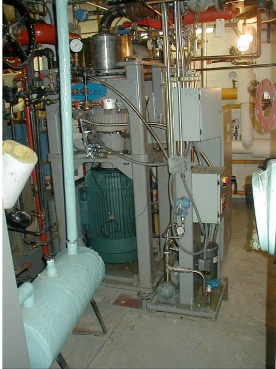
Figure 3 Dual Pressure Euler Turbine During Operation at Rolex Building
