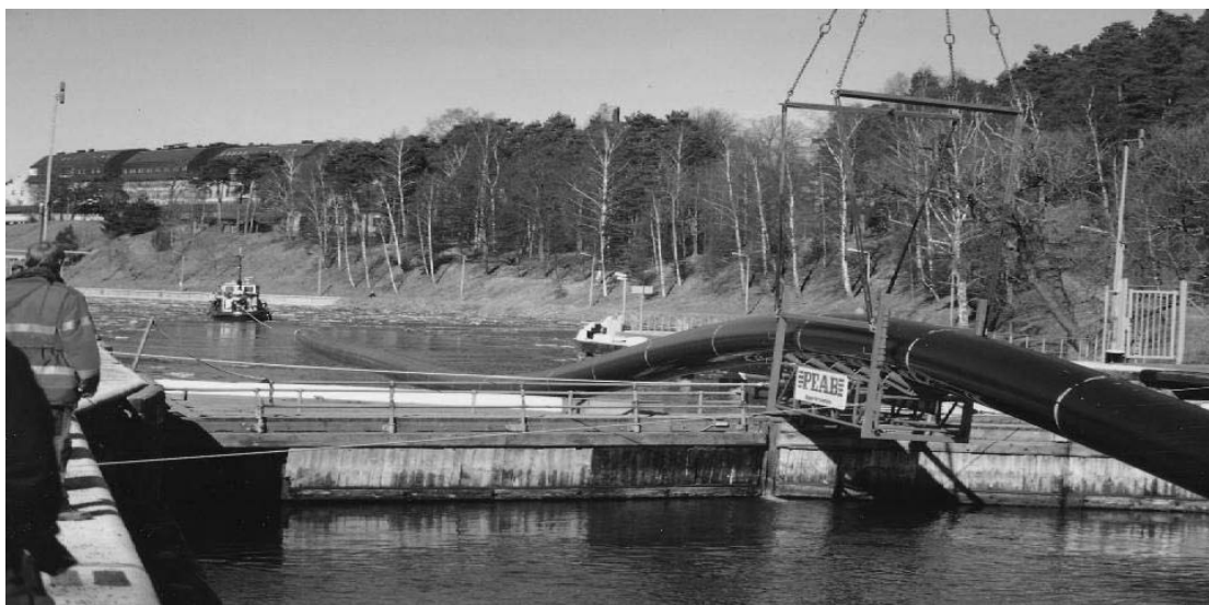
Figure 35. Pipe Installation in Lake Mälaren, Sweden
