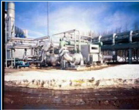
Heat Recovery - Pipelines
