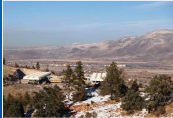
Geothermal Power Plants
